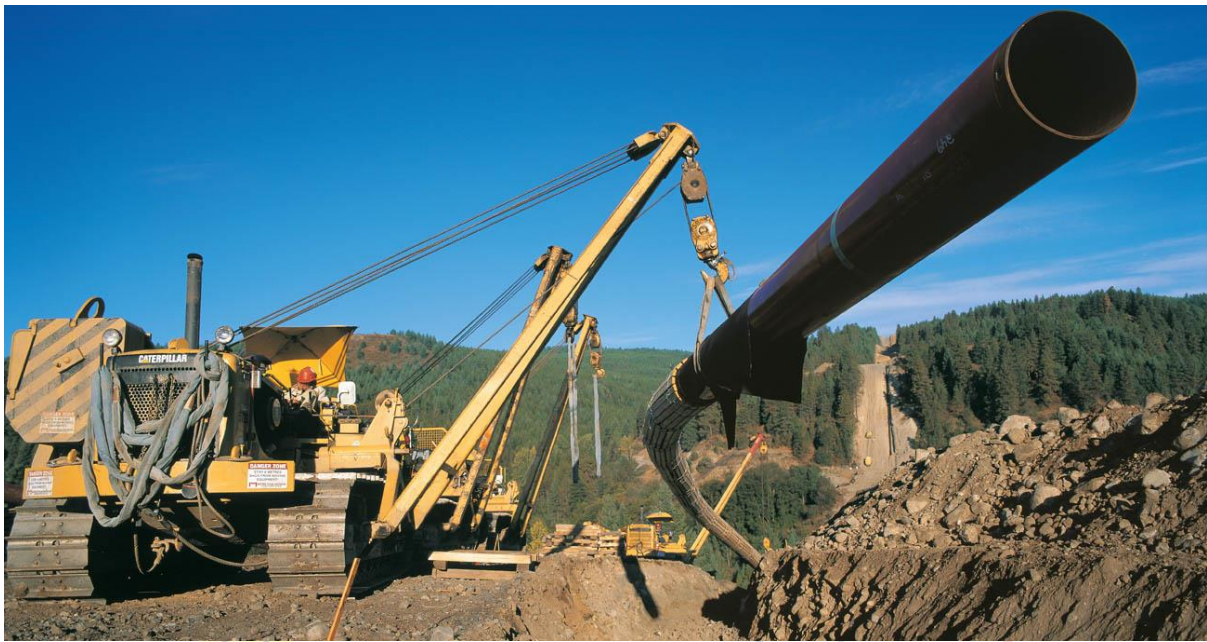
On shore Pipeline Installation
