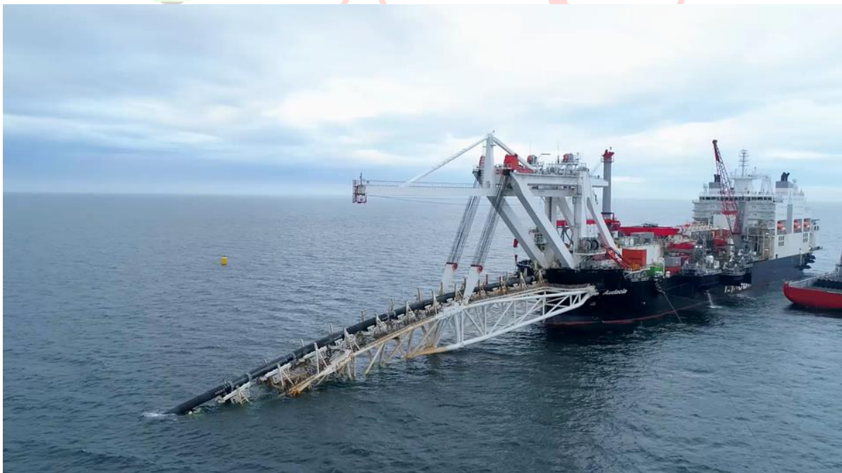
Offshore Pipeline Installation
